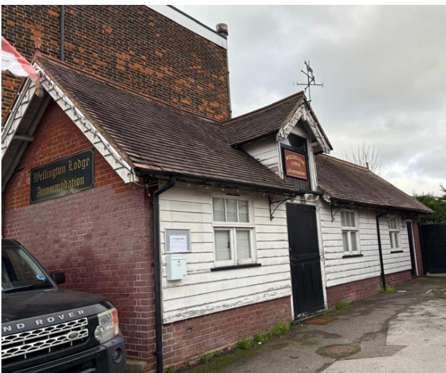
Detached former stables to side
