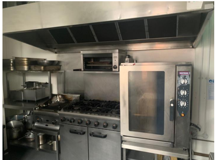
First floor kitchen
