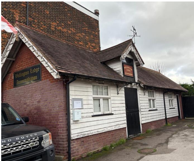
Detached former stables to side
