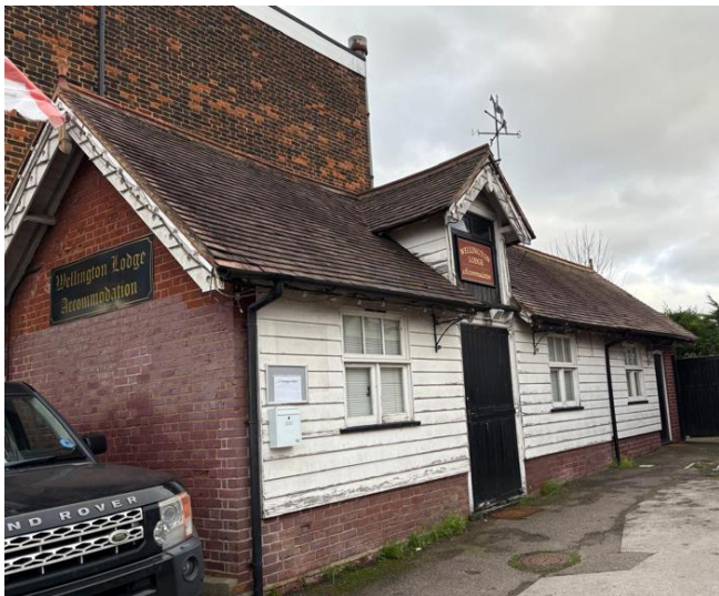
Detached former stables to side
